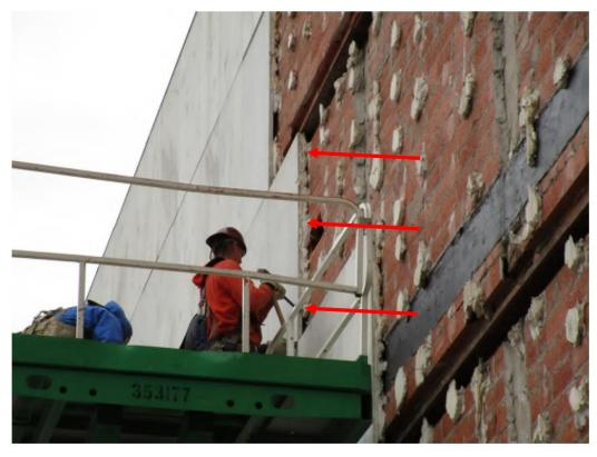
**Photo 1 –** Edge of marble condition, arrows indicate where the copper tiebacks are approximately located at.
