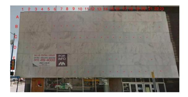
**Photo 2** – Overall view of marble wall with recording grit overlaid onto the elevation. Asterisks represent potential panels which do not match original construction and appear have been replaced for unknown reasons.
