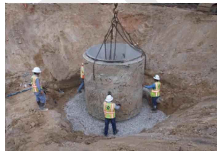
PL19TX Installation of access manway vault at Crossroads Dr.
