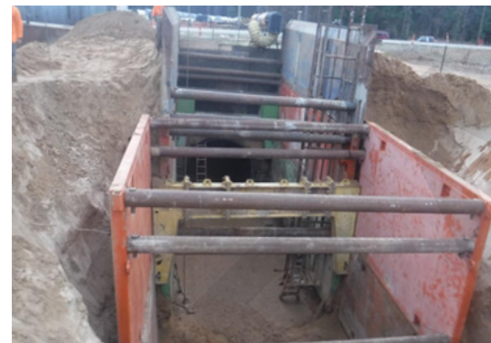
PL19TX Completion of launch shaft extension at SH 19
