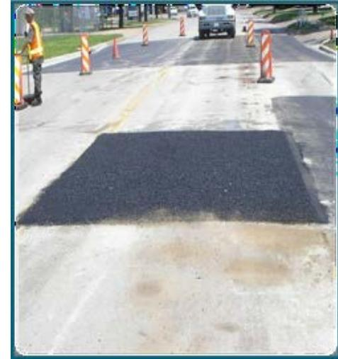
**Slurry Seal** - This treatment for CONCRETE STREETS WITH ASPHALT SURFACE consists of a ¼-inch layer of sand and fine stone mixed with asphalt emulsion. This seals and smooths the surface and conceals scars from previous repairs. It is used predominately for residential roads with curb and gutter. The work is outsourced to a specialized contractor – after Street Services performs preparation work (such as minor base repair and crack sealing).
