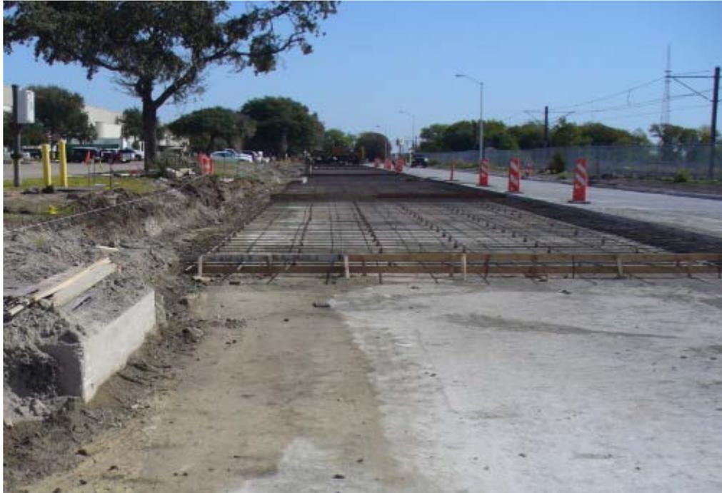
**Reconstruction** - This process is the removal of an existing street with extensive failures and/or badly deteriorated condition. In the process, the pavement is broken and removed (and often recycled), as is the base. Drainage concerns are addressed with this process. The sub-base may be reconditioned as needed, then a new base is placed and compacted. The new concrete surface pavement is then placed, as shown above. The construction work is outsourced under bond-issued funding.
