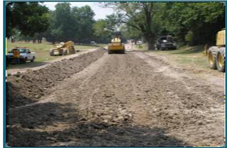
**Rehabilitation** - A treatment for ASPHALT STREETS when a large portion of the surface and the base have deteriorated to an unsatisfactory level. It includes the full-depth repair of base failures, followed by a chip seal, and a new two-inch layer of hot mix asphalt placed over the entire treated segment. Candidate streets are predominately residential asphalt surfaced streets without curb and gutter. **Cost:** \$160K per lane-mile. **Life:** 10-12 years.
