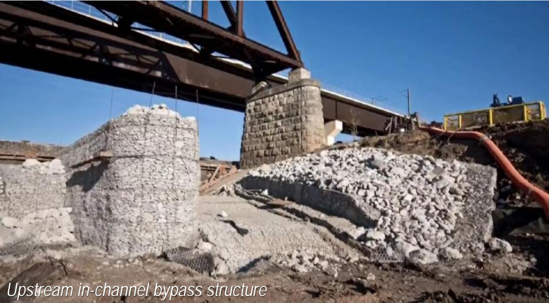
*Upstream in-channel bypass structure*
