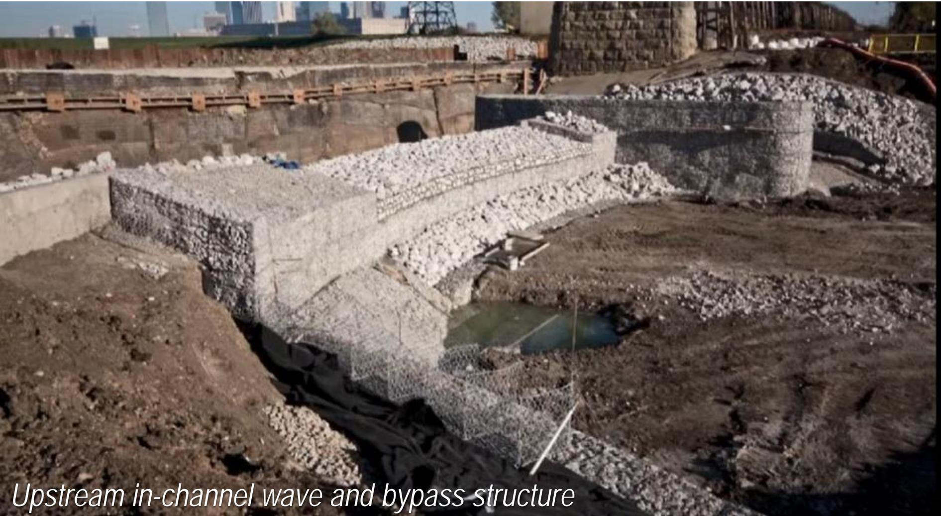
*Upstream in-channel wave and bypass structure*
