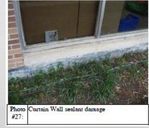
Photo #27: Curtain Wall sealant damage
