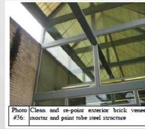
Photo #36: Clean and re-point exterior brick veneer mortar and paint tube steel structure
