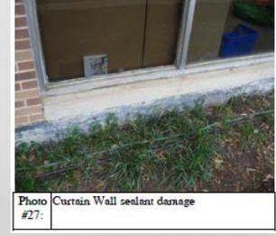
Photo #27: Curtain Wall sealant damage
