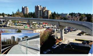
Sound walls can be built into tracks in an aesthetically appealing way while also minimzing sound impacts
