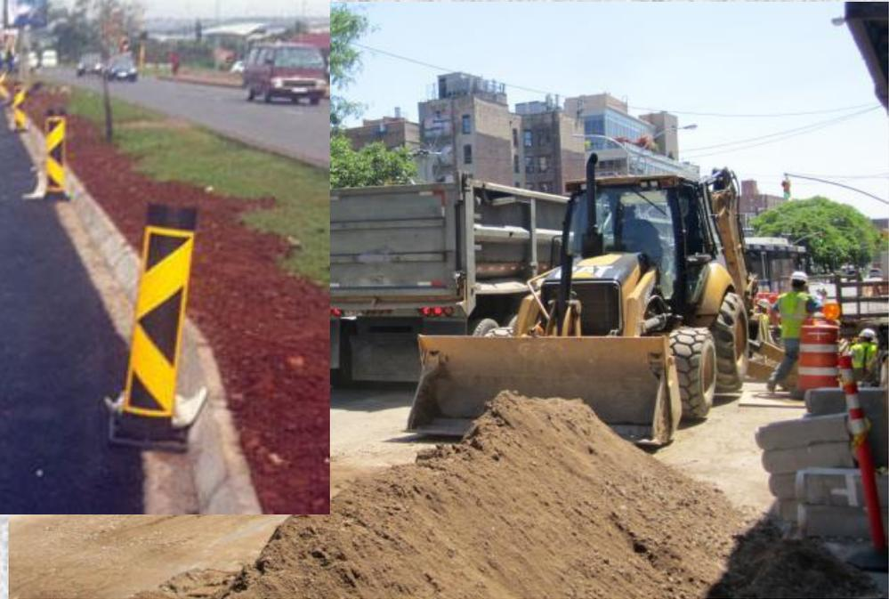
Street and alley repairs by the Dallas Water Utilities are associated with pipeline replacement. For asphalt streets the City policy requires that an entire lane be reconstructed at the location for where the pipeline is replaced. From joint to joint for concrete streets.
