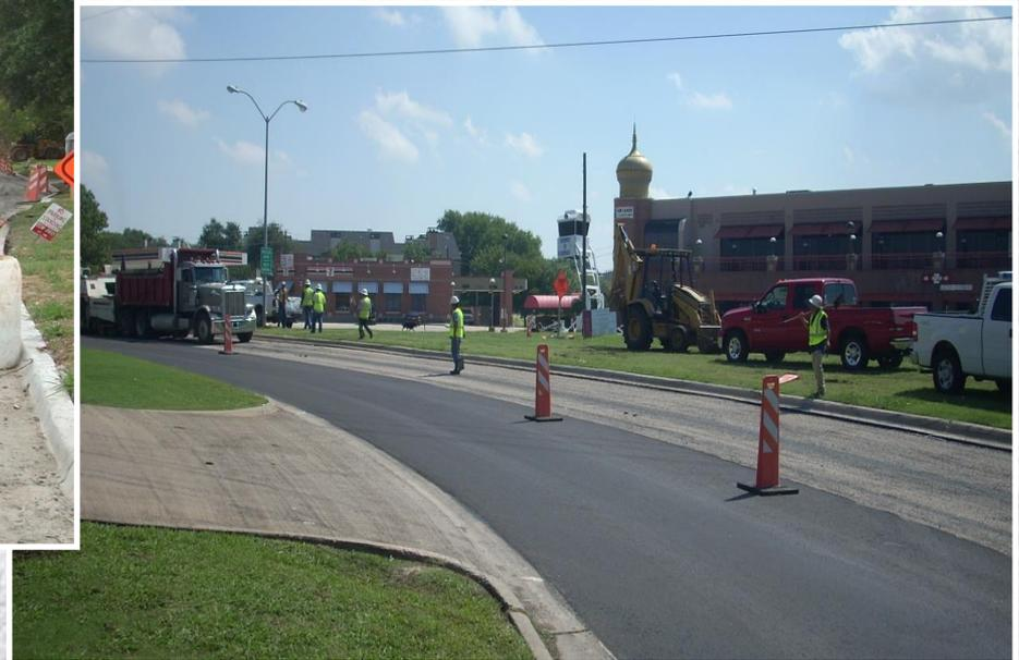
**Re-Surfacing** – This treatment removes the entire asphalt surface, and pulverizes and recycles the old material with new asphalt binder. The new asphalt surface is then placed over the entire surface, compacted, and smoothed to a proper finish. Curb and gutter repair, if needed, is accomplished with the re-surfacing efforts.
