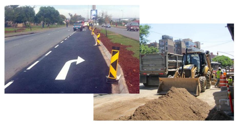
Street and alley repairs by the Dallas Water Utilities are associated with pipeline replacement. For asphalt streets the City policy requires that an entire lane be reconstructed at the location for where the pipeline is replaced. From joint to joint for concrete streets.
