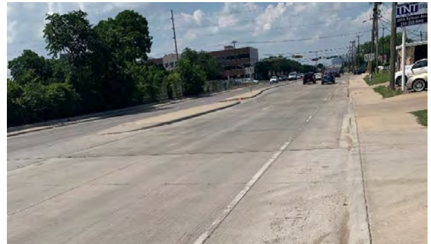
Sylvan Ave. (North of Singleton Blvd. looking North)
