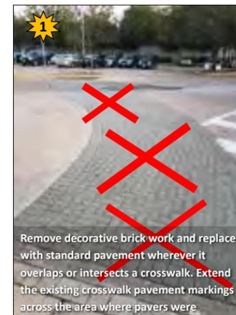
Remove decorative brick work and replace with standard pavement wherever it overlaps or intersects a crosswalk. Extend the existing crosswalk pavement markings across the area where pavers were
