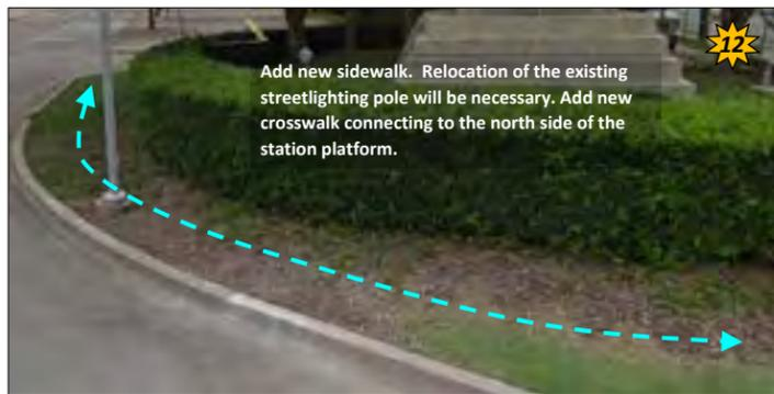
Add new sidewalk. Relocation of the existing streetlighting pole will be necessary. Add new crosswalk connecting to the north side of the station platform.
