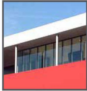
Point supported guard rail. 38% coverage of North Elevation.
