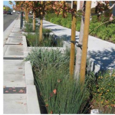
New rain gardens around existing trees on sidewalk capture runoff water from the street and sidewalk.
