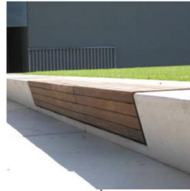
New poured-in-place concrete benches along sidewalk are incorporated into Radiator Plaza plinth.
