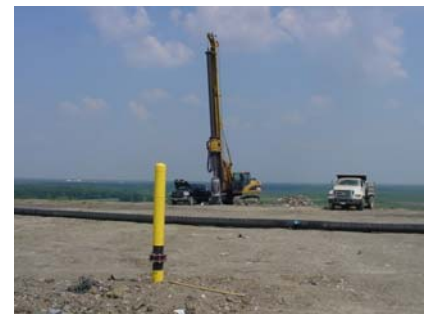
Drilling Gas Well -photograph by Adam Jochelson
