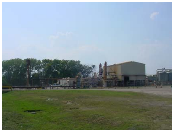
Gas Processing Plant
