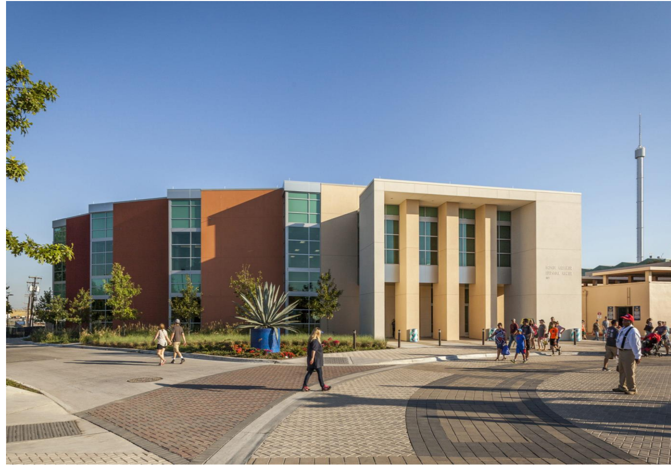
Briscoe Carpenter Exterior
