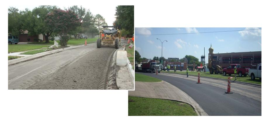
**Re-Surfacing** – This treatment removes the entire asphalt surface, and pulverizes and recycles the old material with new asphalt binder. The new asphalt surface is then placed over the entire surface, compacted, and smoothed to a proper finish. Curb and gutter repair, if needed, is accomplished with the re-surfacing efforts. **Cost:** \$200K per lane-mile. Life: 15-20 years (with maintenance).
