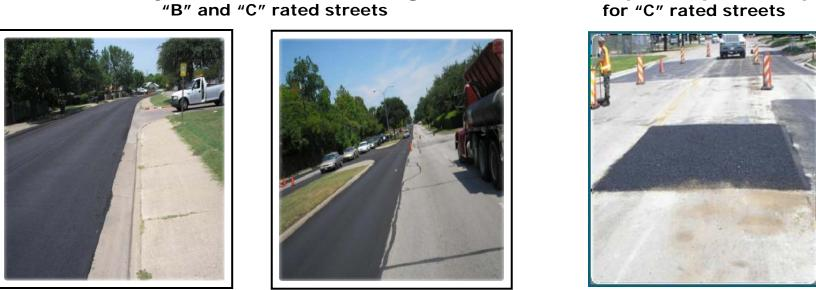
**Slurry Seal** - This treatment for CONCRETE STREETS WITH ASPHALT SURFACE consists of a ¼-inch layer of sand and fine stone mixed with asphalt emulsion. This seals and smooths the surface and conceals scars from previous repairs. It is used predominately for residential roads with curb and gutter. The work is outsourced to a specialized contractor – after Street Services performs preparation work (such as minor base repair and crack sealing). **Cost:** \$13K per lane-mile. Life: 5-7 years.
