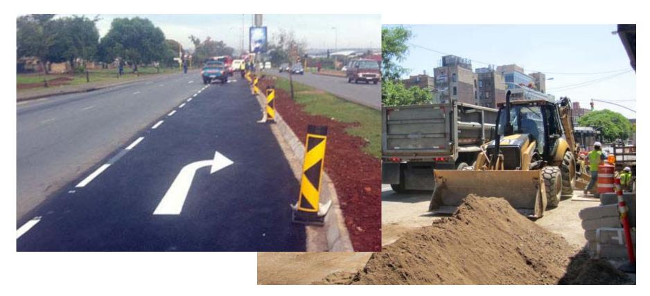
Street and alley repairs by the Dallas Water Utilities are associated with pipeline replacement. For asphalt streets the City policy requires that an entire lane be reconstructed at the location for where the pipeline is replaced. From joint to joint for concrete streets. 24
