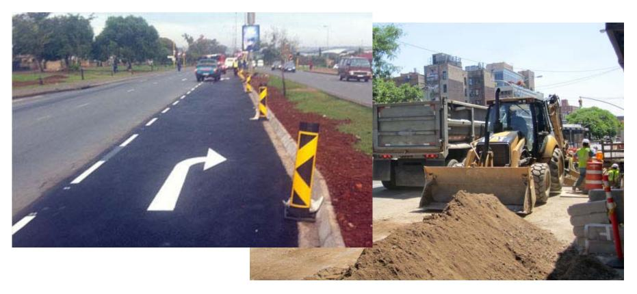
Street and alley repairs by the Dallas Water Utilities are associated with pipeline replacement. For asphalt streets the City policy requires that an entire lane be reconstructed at the location for where the pipeline is replaced. From joint to joint for concrete streets.
