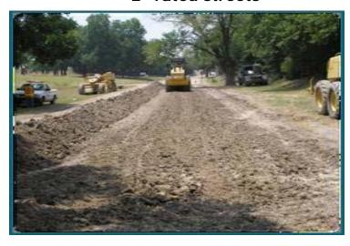
**Rehabilitation** - A treatment for ASPHALT STREETS when a large portion of the surface and the base have deteriorated to an unsatisfactory level. It includes the full-depth repair of base failures, followed by a chip seal, and a new two-inch layer of hot mix asphalt placed over the entire treated segment. Candidate streets are predominately residential asphalt surfaced streets without curb and gutter. **Cost:** \$160K per lane-mile. **Life:** 10-12 years.
