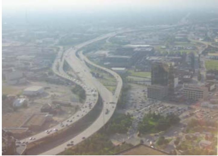
Figure 9 - Stemmons Freeway as seen from Downtown
