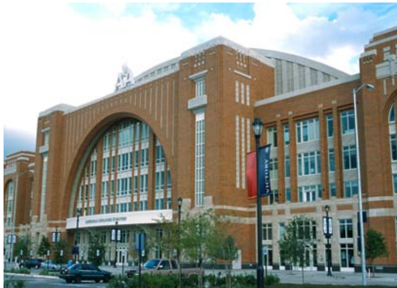
Figure 3 - The American Airlines Center is an anchor of the Victory Development area, home to hotels, restaurants, and multifamily residential development all in a walkable urban environment served by the DART light rail system.
