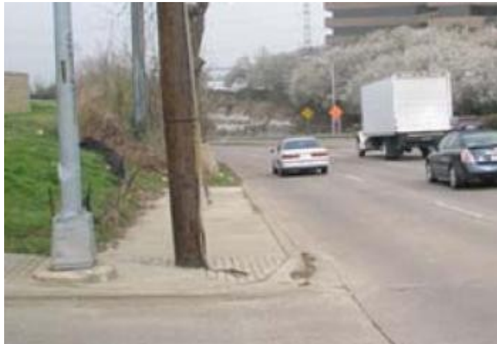
Figure 10 - Utilities and the Pedestrian Environment. Utility transmission lines and poles in the right-of-way can hinder a quality pedestrian environment.
