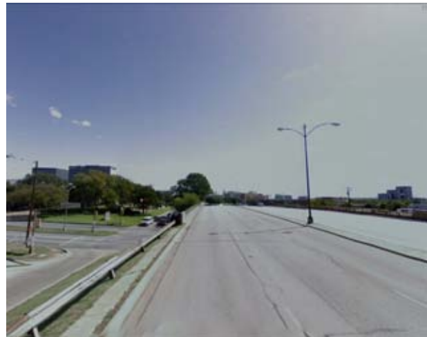
Figure 38 - Facing south on Harry Hines Boulevard crossing over Mockingbird Lane. This one of the northern entry points into the Southwestern Medical District.
