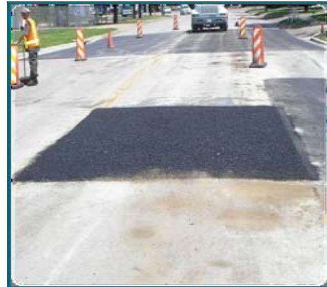
Full-Depth Asphalt Repair
