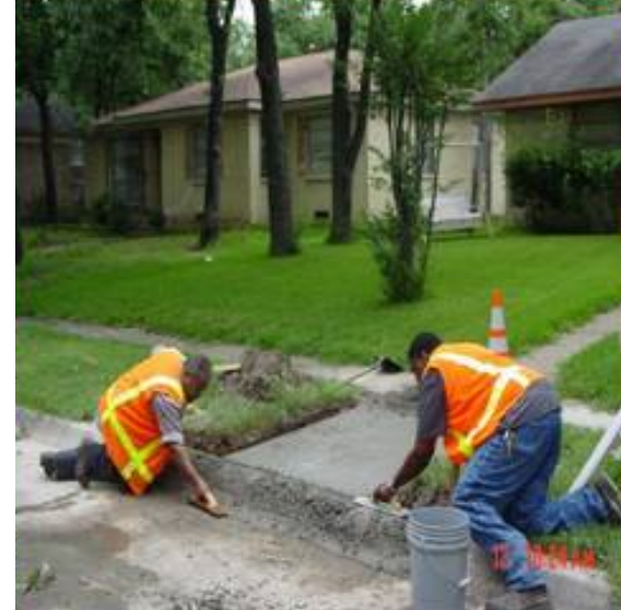
Curb and Gutter w/Sidewalk
