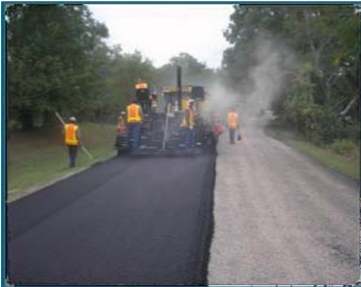
Street Overlay (Rehabilitation/Restoration)
