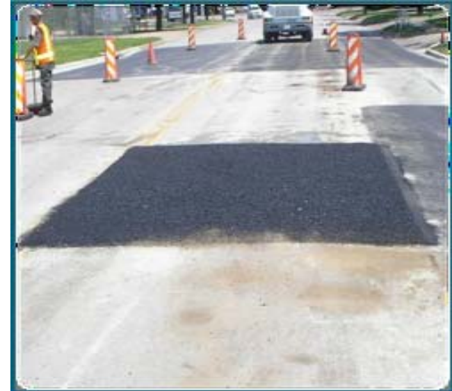
Full-Depth Asphalt Repair
