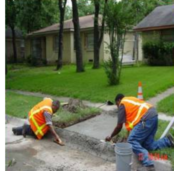
Curb and Gutter w/Sidewalk
