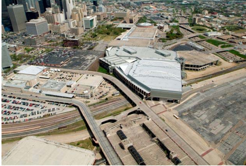
Figure 4. Aerial View of the Dallas Convention Center and Surrounding Area
