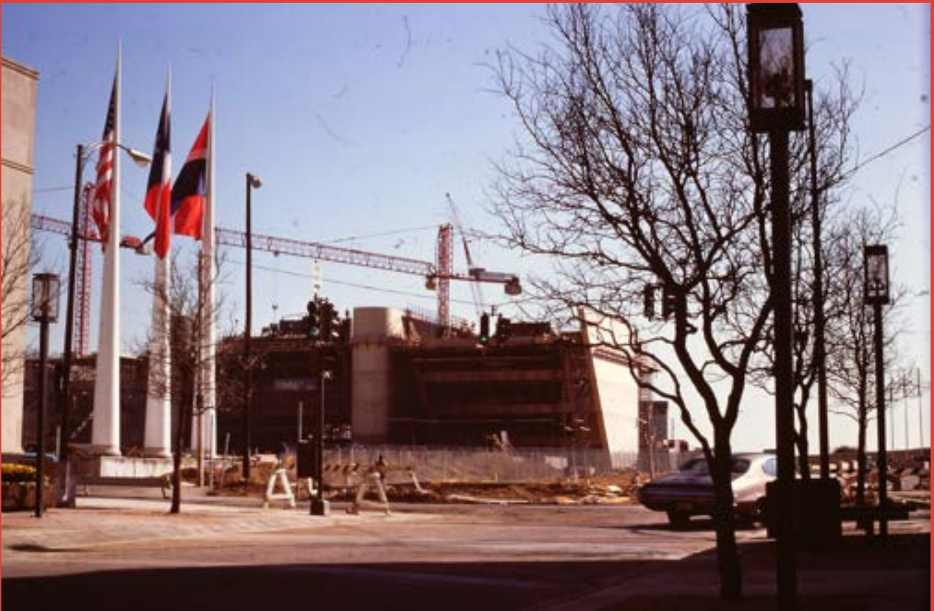
City Hall under construction, 1974. Image courtesy of the City of Dallas historic preservation team.
